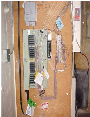
Existing Telephone Wiring Termination Installation
