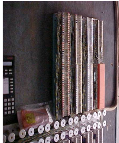
New Telephone Wiring Termination Installation
