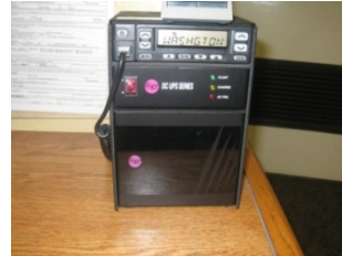
Secondary School New Base Station
